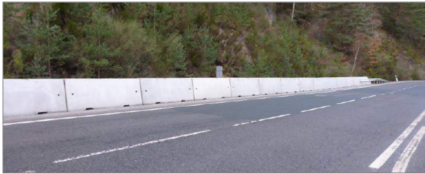
Precast concrete New Jersey barriers
