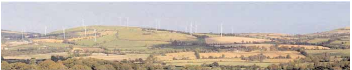
2(c) Wind energy development with random layout - this response is inappropriate given the patchwork field pattern of this landscape.
