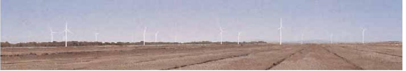
3(a) Random layout - the random spacing is not entirely appropriate to the simplicity of this landscape.
