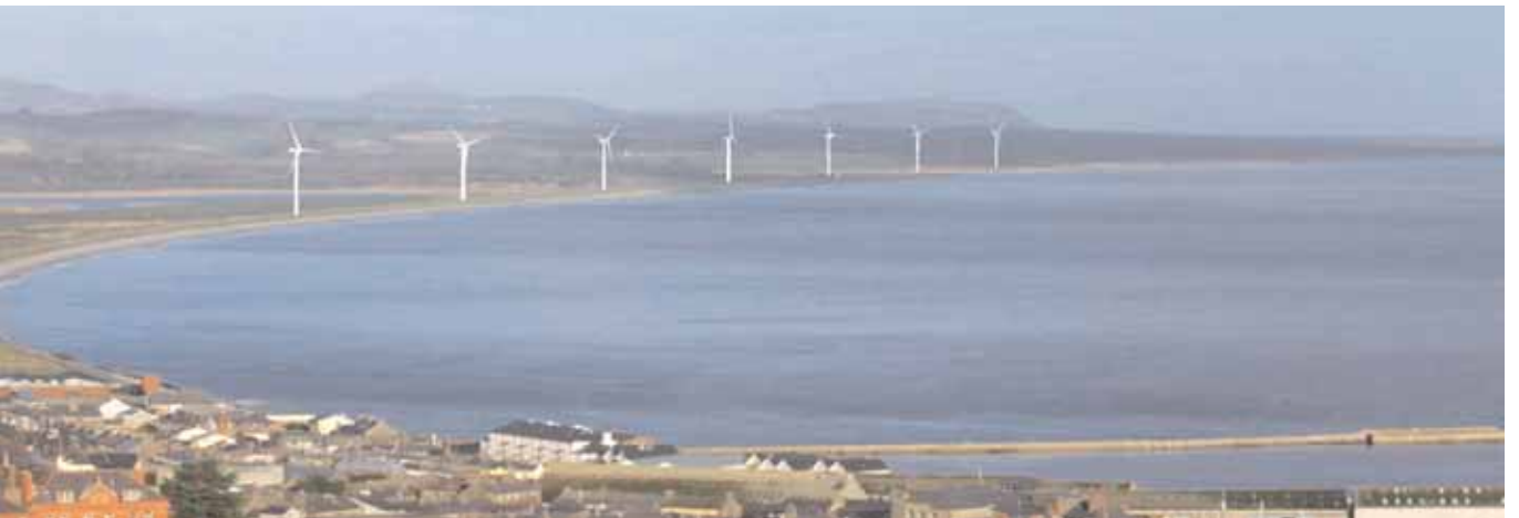
6(d) Wind energy development with simplicity involving regular spacing, a linear layout and level profile is usually preferable.
