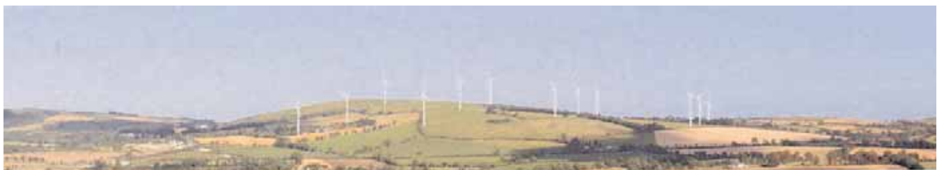
2(d) Wind energy development with grid layout - this response involving any form of linear layout and regular spacing is appropriate given the patchwork field pattern of this landscape.
